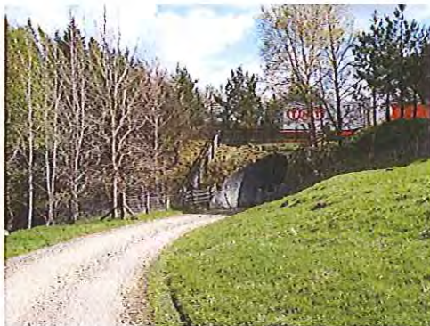
Fig. 7 : Access track emerging from underpass
